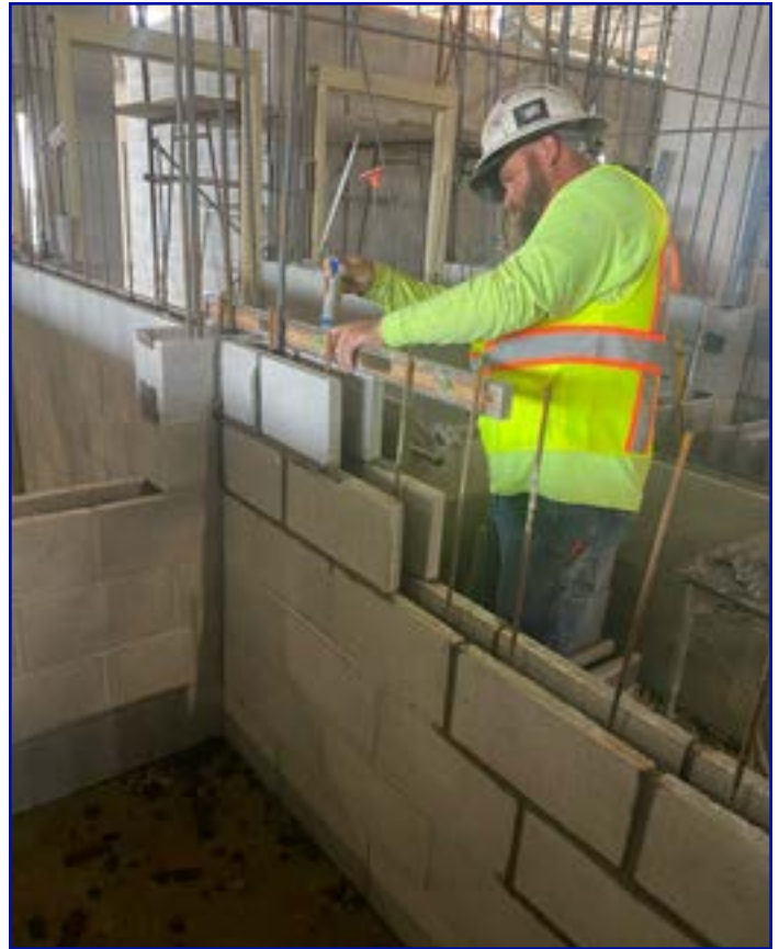
New Member John Porter with Bratton Masonry at the Modesto Courthouse.
