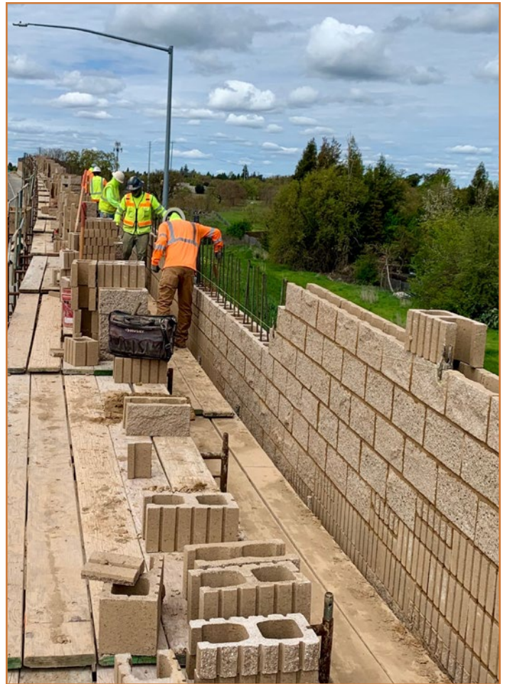
PTS Masonry I-5 Soundwall
