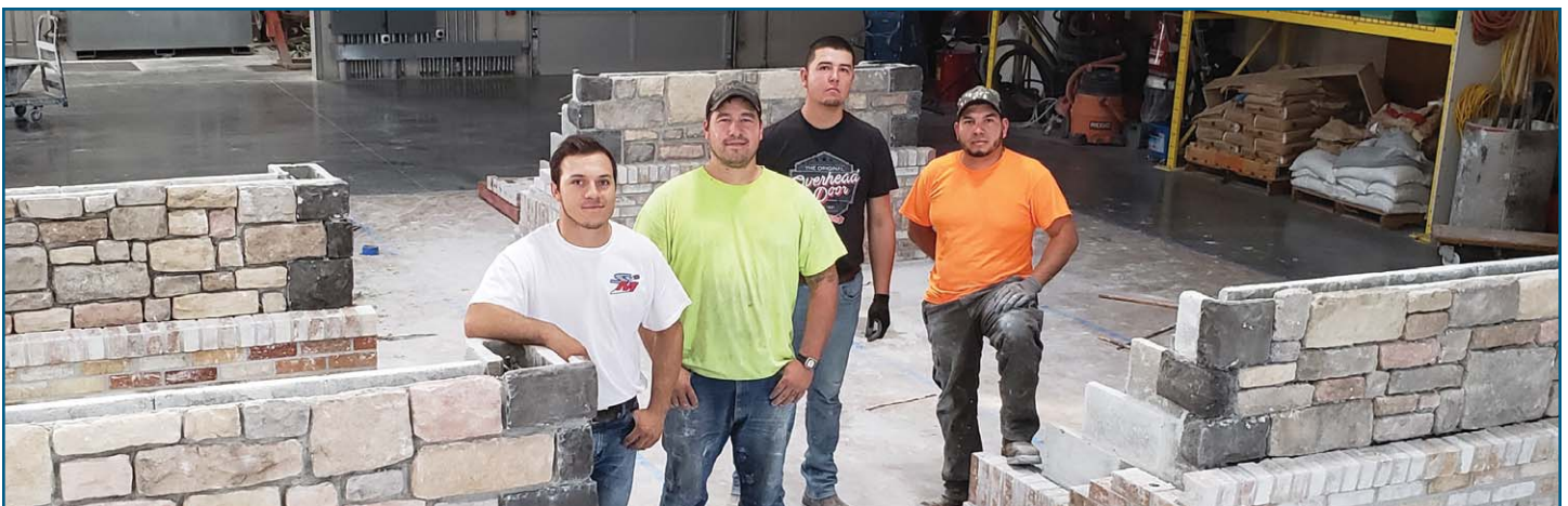
Brick Class 4-CMU wall with reinforcement, brick veneer with soldier and projecting rolok sill, and cultured stone veneer. From Left: Mason Temple (Stoney Masonry), Ken Powell (John Jackson Masonry), Mario Montano (Patania Masonry), and Adan Cornejo (Cornerstone Masonry).
