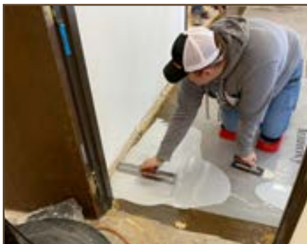
Brian Dohring spreading crack isolation membrane.
